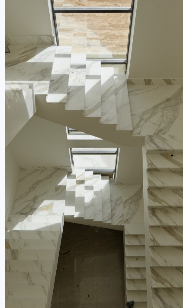
Interior Staircase Skylight Glazing
