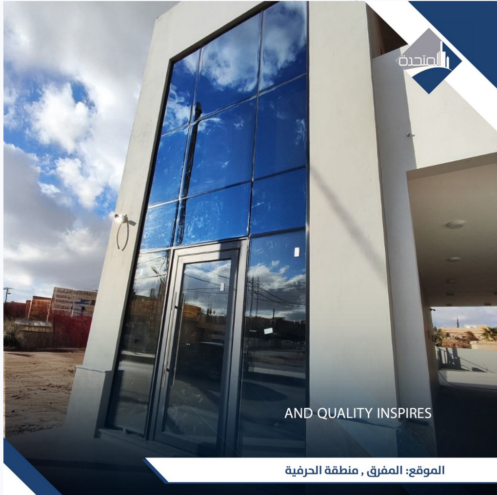
Glass Curtain Wall Entrance — Al-Mafraq
